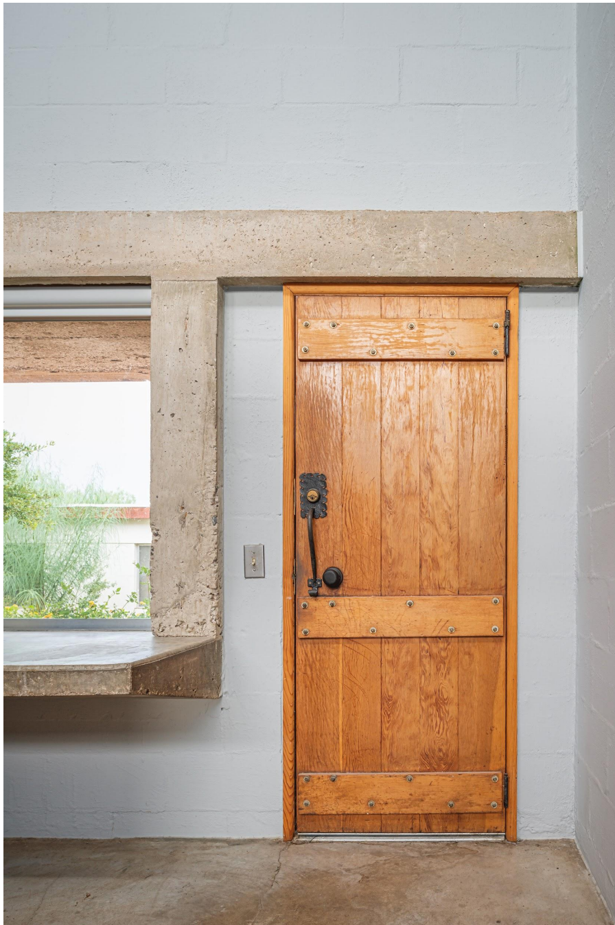
Fig. 10, South door with exposed structural concrete and painted concrete block.
