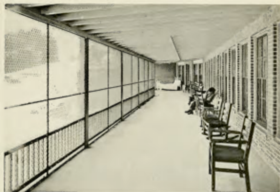
No. 32.—Eastern Maine Hospital, Bangor, Me. T. C. & J. H. STEVENS, ARCHITECTS. ILLUSTRATING A METHOD OF PROTECTING A SLEEPING PORCH WITH HEAVY WIRE NETTING. USEFUL WHEN A PORCH FACES A STREET OR TO PREVENT PATIENTS FROM LEAVING WITHOUT PERMISSION.
