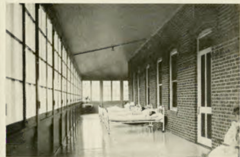
No. 33.—United States Hospital for the Insane, Washington, D. C. SHOWING A METHOD OF INCLOSING A SLEEPING PORCH WITH SWINGING SASH FRAMES; USEFUL FOR CITY HOSPITALS WITH PORCHES HAVING VARIOUS EXPOSURES.
