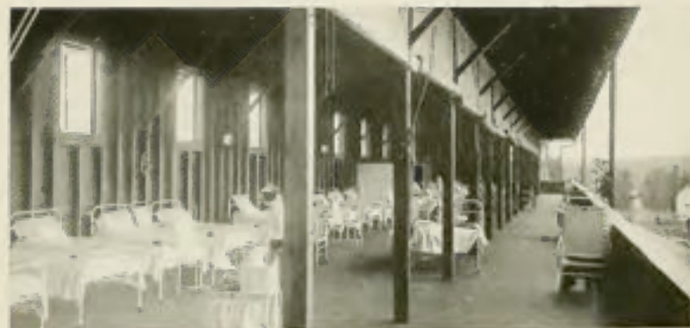
No. 71.—Virginia State Farm, Richmond, Va. VIEW OF OPEN PORCH ILLUSTRATING MANNER OF PROTECTING PORCHES BY CANTAS CURTAINS PLACED BETWEEN PILLARS, A FEW FEET BACK FROM THE LINE OF THE ROOF PROJECTION.
