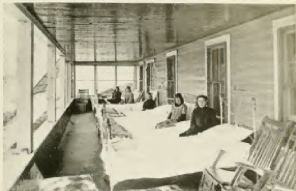
No. 72.—Loomis Sanatorium, Liberty, N. Y. VIEW OF CHAPMAN COTTAGE, SLEEPING PORCH; ILLUSTRATING METHOD OF CONSTRUCTION AND INTERIOR FINISH, USING NARROW FLOOR BOARDS FOR SEALING. (See illustrations 1, 73, 92 and 105 for further descriptions of this institution.)
