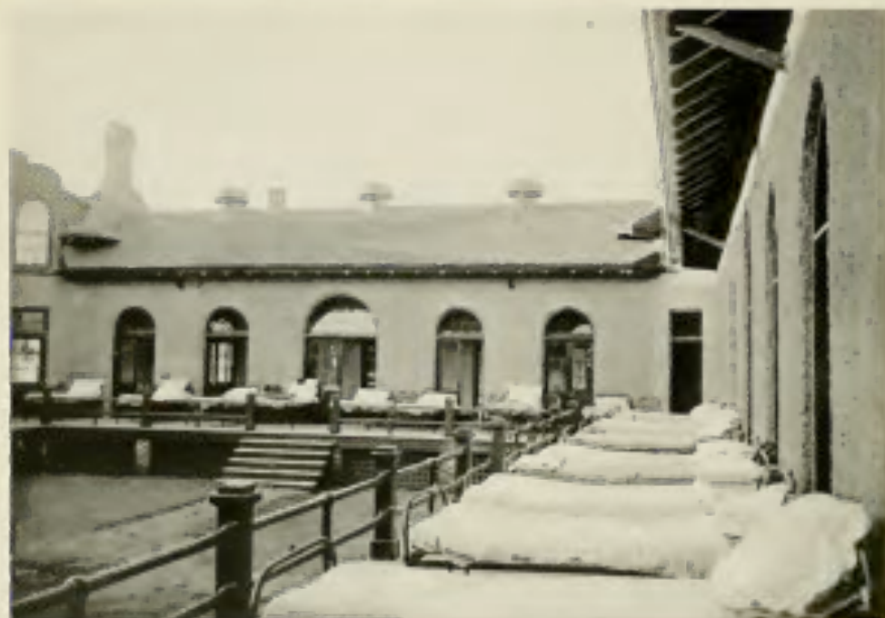
No. 35.—United States Army General Hospital, Fort Bayard, N. M. VIEW OF INNER COURT SHOWING SLEEPING PORCHES.
