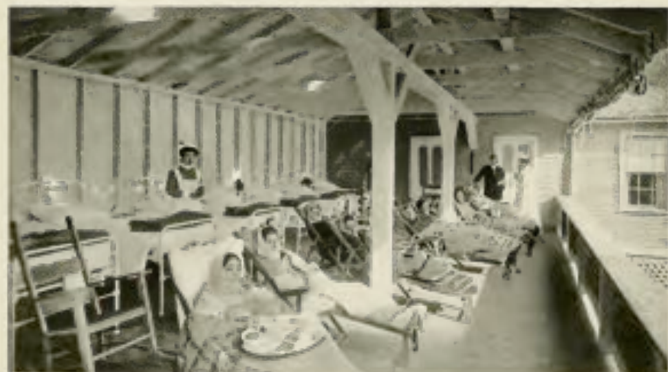
No. 69.—Catawba Sanatorium, Catawba, Va. DESIGNED BY DR. ELLISON G. WILLIAMS. VIEW OF AN OPEN PORCH ILLUSTRATING A METHOD OF CONSTRUCTION WITHOUT INTERIOR FINISH, AND A MANNER OF PROTECTING PORCHES BY CANVAS CURTAINS UNDER THE EDGE OF THE ROOF PROJECTION. (See illustrations 17, 30 and 80 for further description of this institution.)
