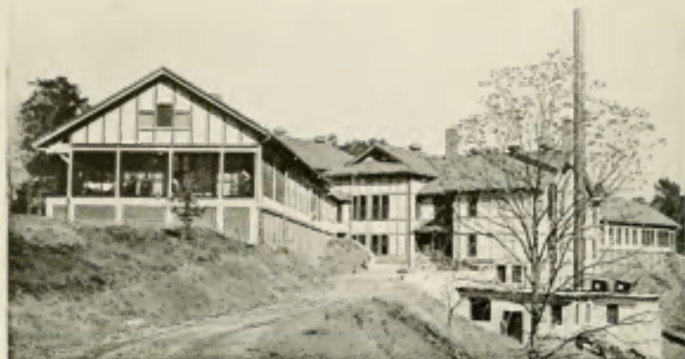
No. 18.—Waverly Hill Sanatorium, Waverly Hill, Ky. J. J. GATSEY, ARCHITECT. VIEW FROM THE REAR SHOWING A METHOD OF USING THE TOP AND SIDE OF A HILL IN ORDER TO OBTAIN A POSITION BELOW THE BUILDINGS FOR THE POWER PLANT. (See illustration 5 for further description of this institution.)
