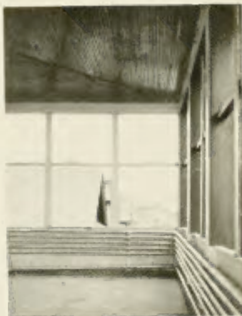
No. 47.—Isolation Hospital, Paterson, N. J. CHARLES E. WHITE, ARCHITECT. VIEW OF THE CORNER OF ONE OF THE PORCHES SHOWING METHOD OF HEATING FOR ADVANCED CASES BY STEAM PIPES. (See illustration 52 for further description of this institution.)
