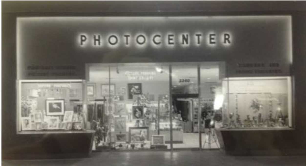
Fig.16, The Chuck Abbott developed Photocenter (1947), Architectural design attributed to Frank Nelson. Tucson Historic Preservation Foundation digital archive.
