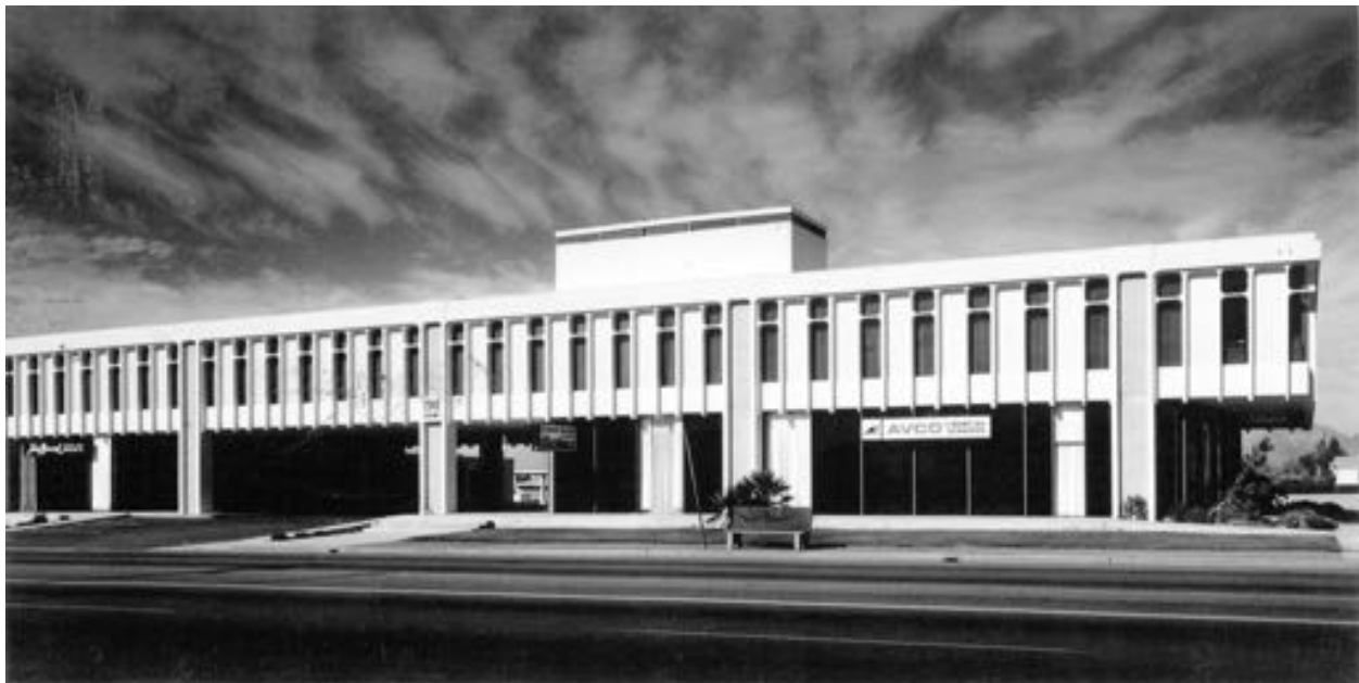
Fig. 30, Kelly Building, Nicholas Sakellar, photo c. 1965.
