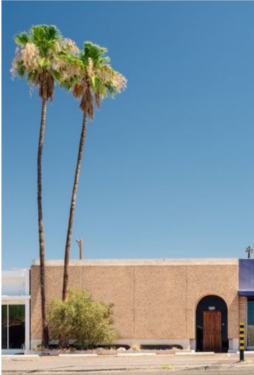
Fig. 18. Friedman Office Building, (1950, 1965 & 1967), Photo by GMVargas 2017.
