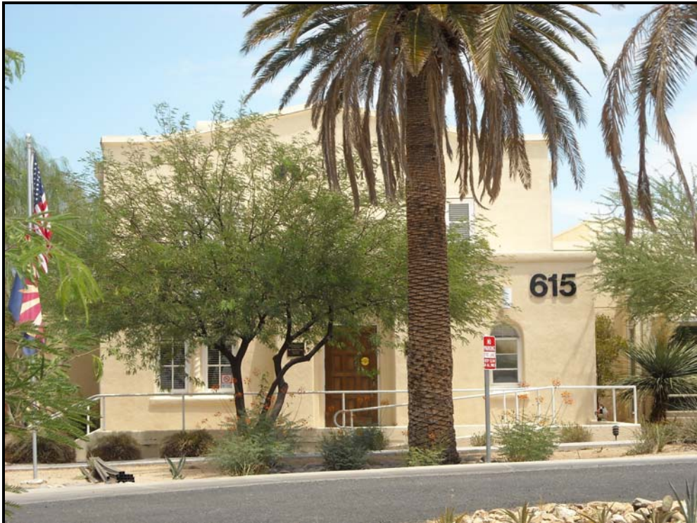
Photograph 7. St. Luke's-In-The-Desert, main administration building, view facing north (2010).
