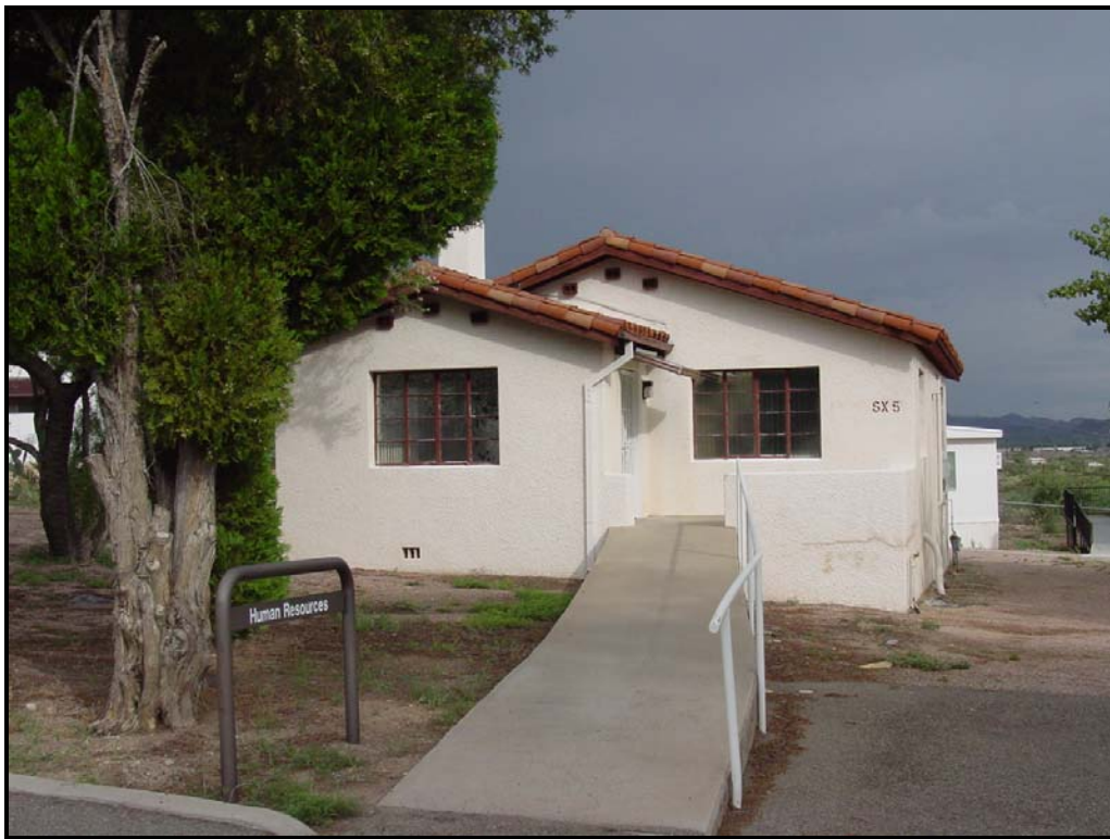
Photograph 41. Former physician residence (San Xavier-5), view facing northwest (2010).
