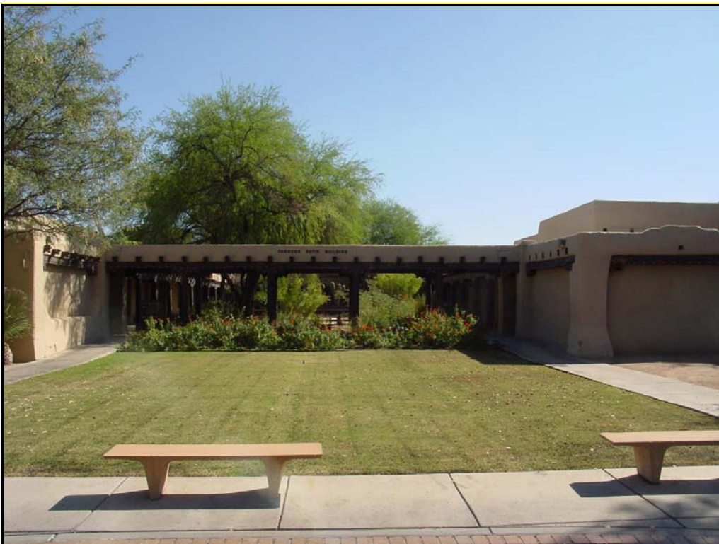
Photograph 15. West elevation of Patio Building (Institute of Medical Research) at the former Desert Sanatorium (now Tucson Medical Center), view facing east (2010).
