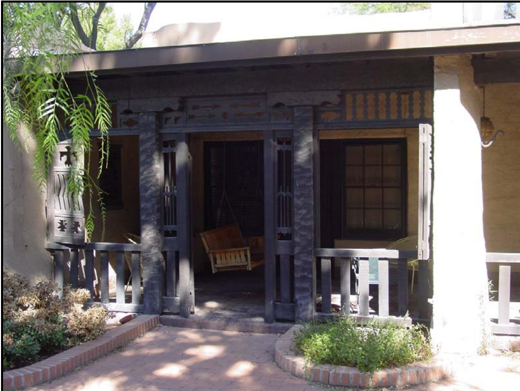
Photograph 23. Detail of porch and south elevation of the Erickson Residence (Desert Sanatorium), view facing northeast (2010).
