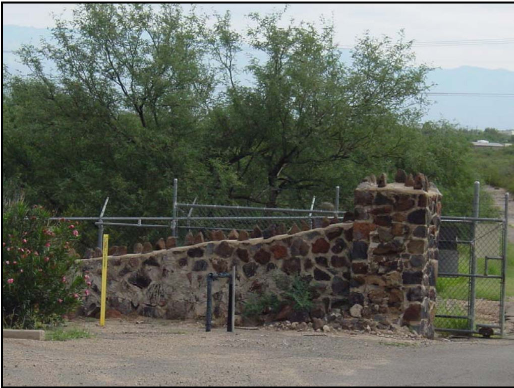
Photograph 46. Volcanic cobble perimeter wall at the former San Xavier Sanatorium, view facing east-southeast (2010).
