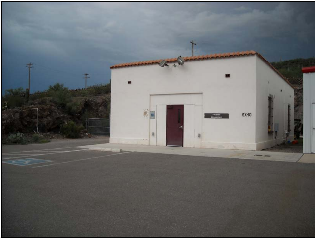
Photograph 45. Former custodial/maintenance warehouse (San Xavier-10), view facing southeast (2010).
