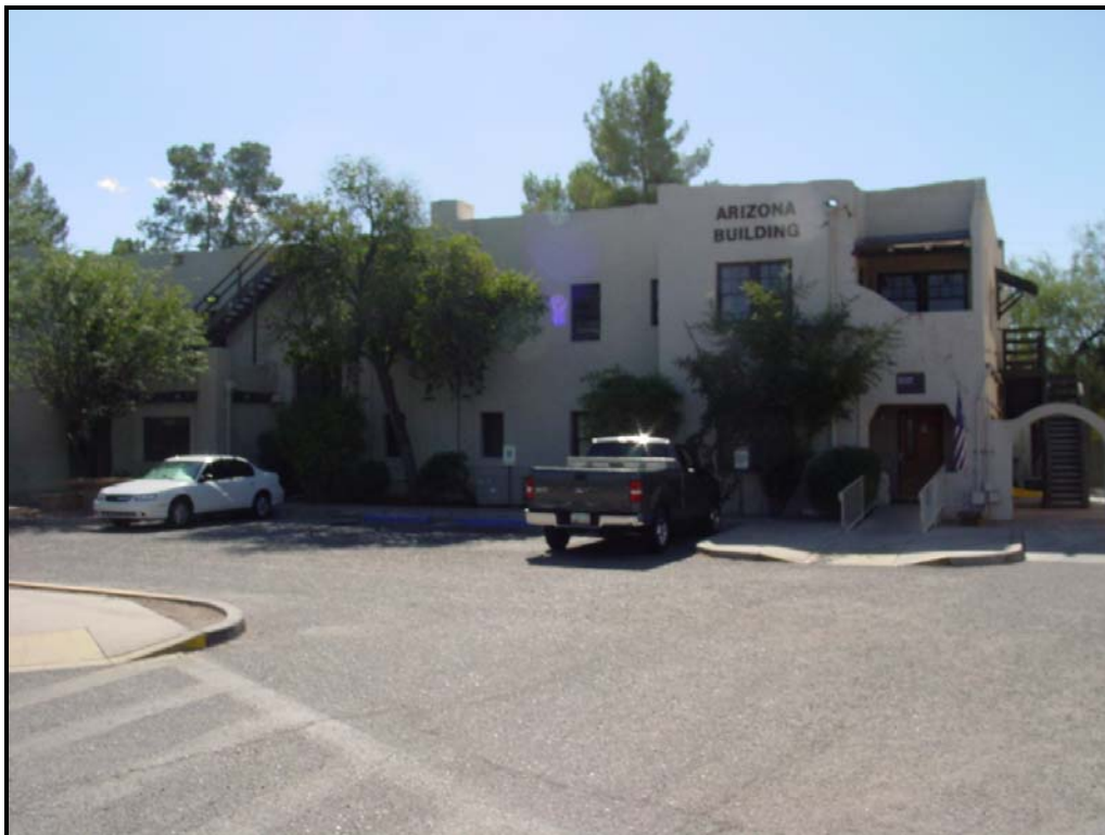
Photograph 18. East elevation of the Arizona Building (nurse's residence) at the former Desert Sanatorium (now Tucson Medical Center), view facing west-southwest (2010).
