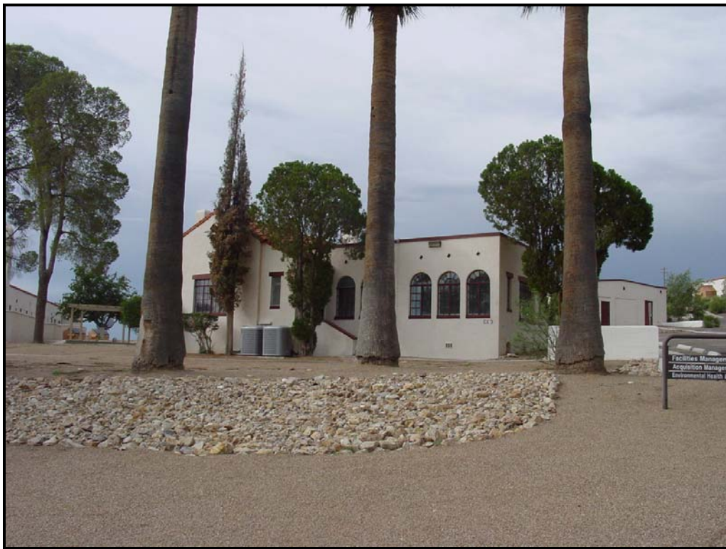
Photograph 39. Former superintendent's residence (San Xavier-3), view facing south-southeast (2010).
