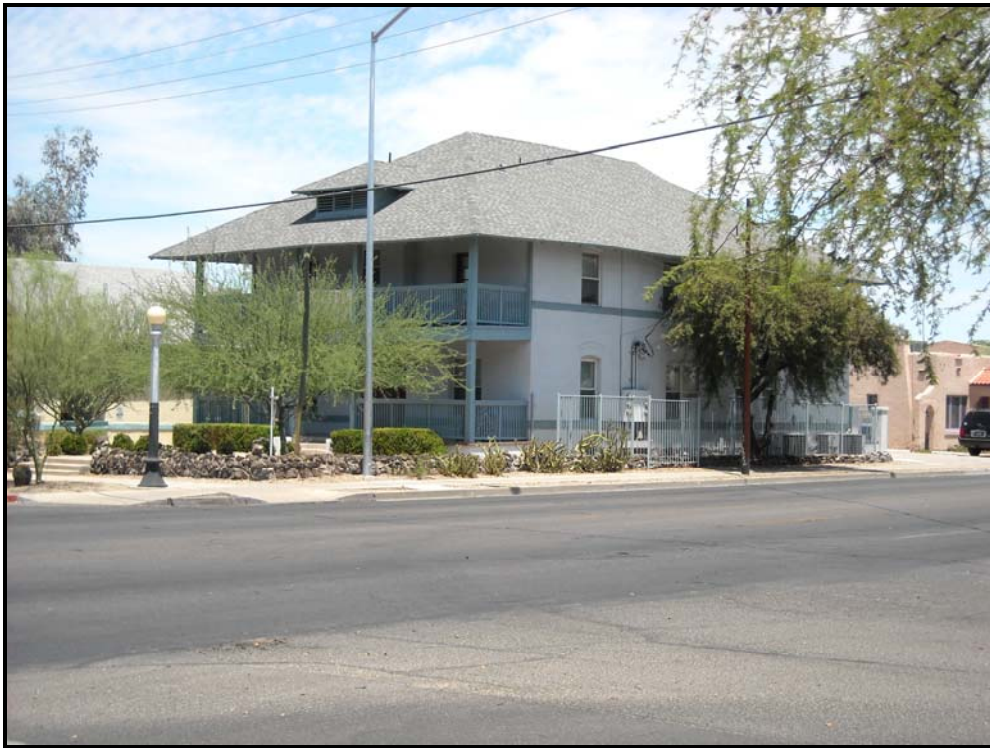
Photograph 11. Carter's Hotel Rest Sanatorium, view facing northwest (2010).
