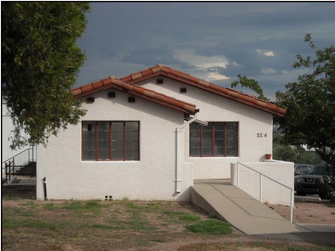
Photograph 40. Former physician housing (San Xavier-4), view facing northwest (2010).
