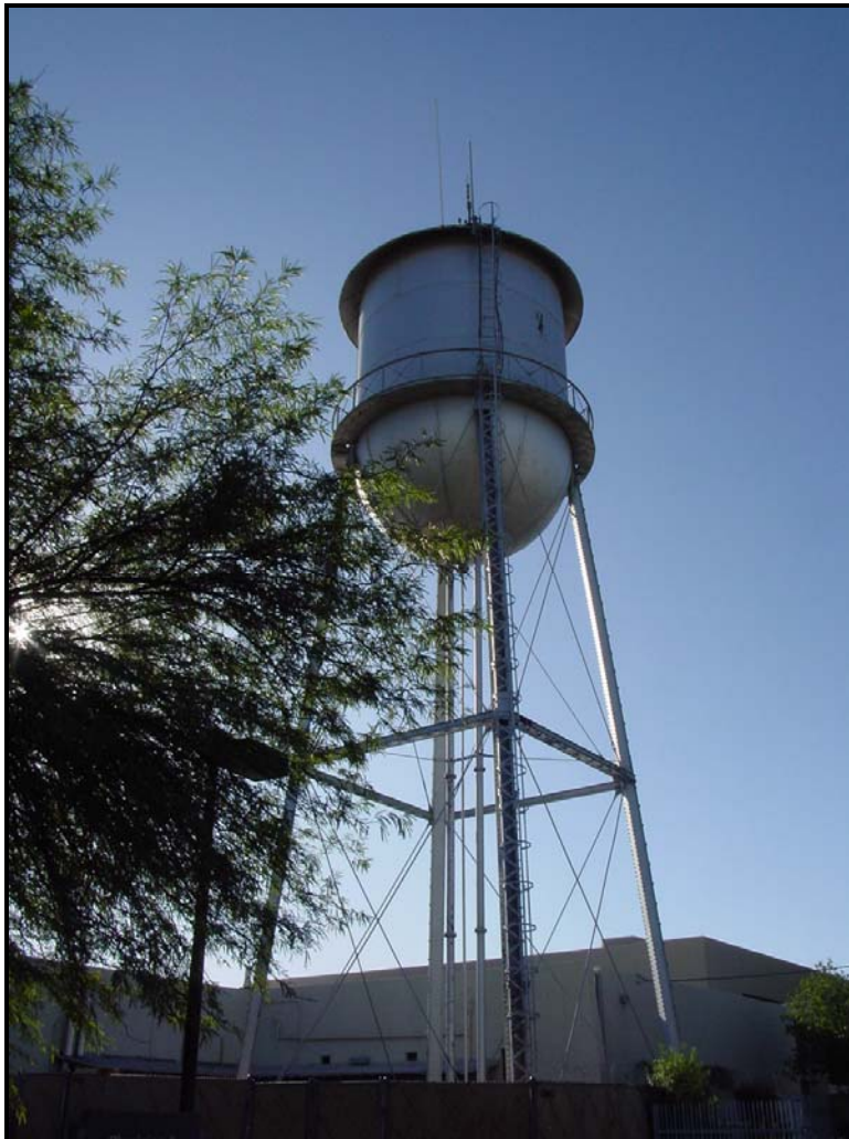
Photograph 24. Water Tower at the former Desert Sanatorium, view facing southeast (2010).
