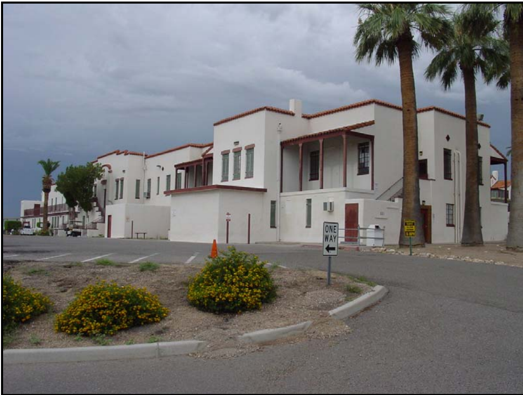
Photograph 37. Main hospital building (SX-1) at the former San Xavier Sanatorium, view facing southeast (2010).
