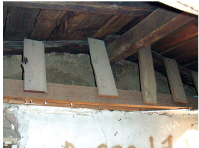
Site-built roof framing in northern rooms
