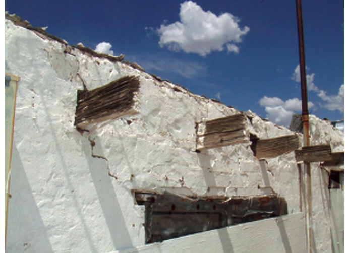
Roof framing at south wall. Note rotted joist ends.
