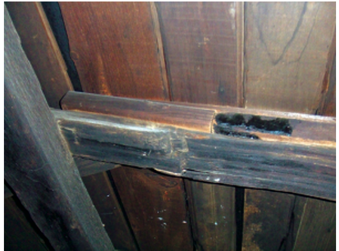
Charred roof framing with additional framing placed on top. This condition exists throughout the northern rooms
