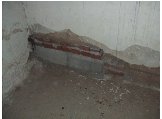
Infill masonry at the base of the eastern wall in the north-central room
