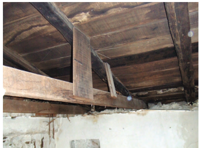
Typical roof framing in northern rooms.
