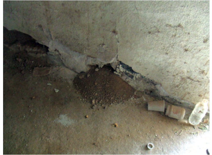
Deteriorated adobe at base of wall caused by burrowing vermin
