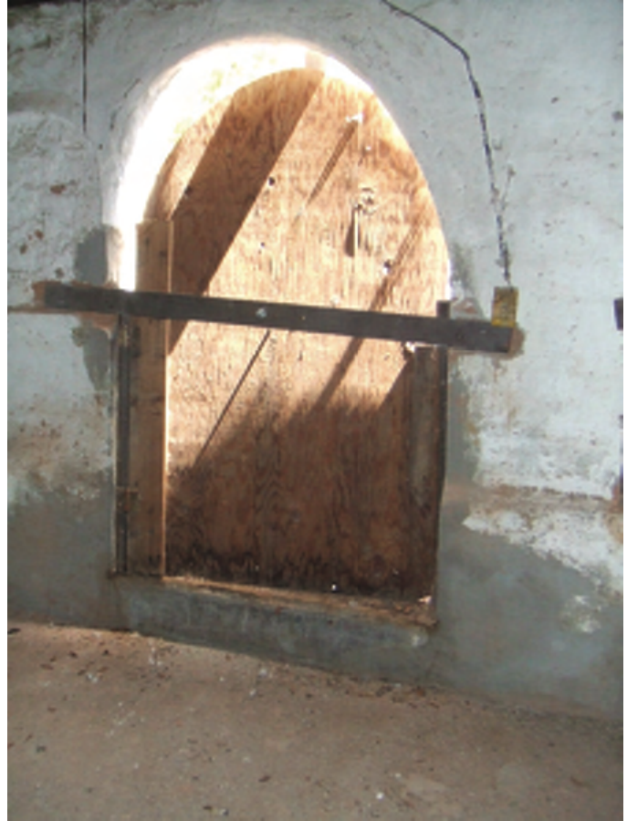
Arched opening at southeastern room
