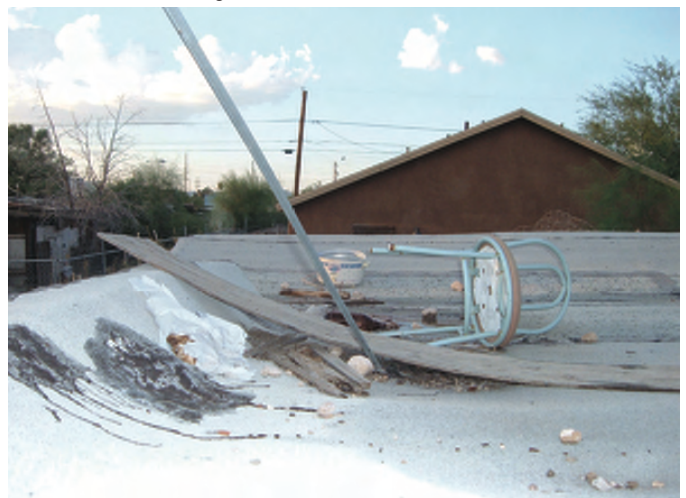
Roof with loose debris
