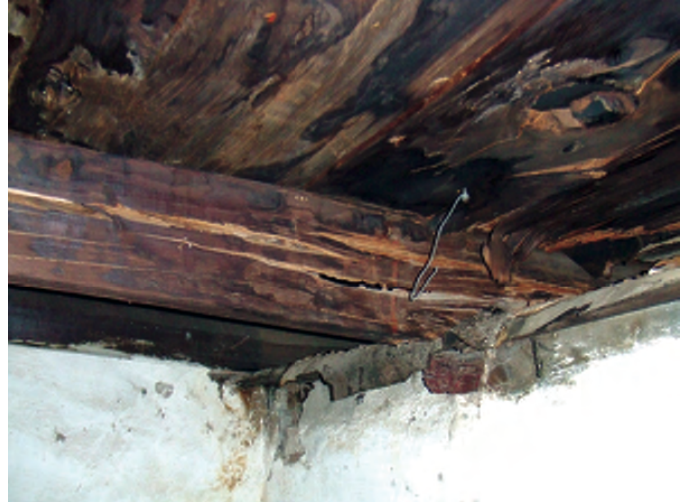
Split roof joist at SW at room in southwest corner. Notice severe water damage to roof decking caused by faulty roof design.
