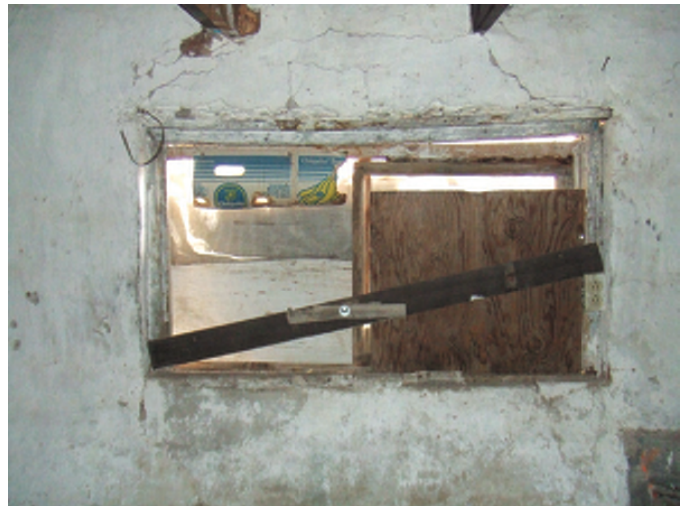
Wood framed window opening at southwest room.
