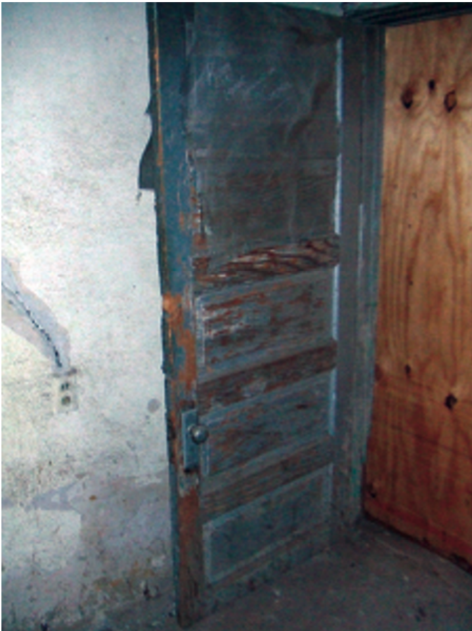
Exterior wood door at north-central room
