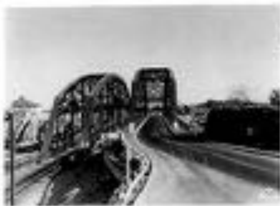
BRIDGE OVER RIVER
