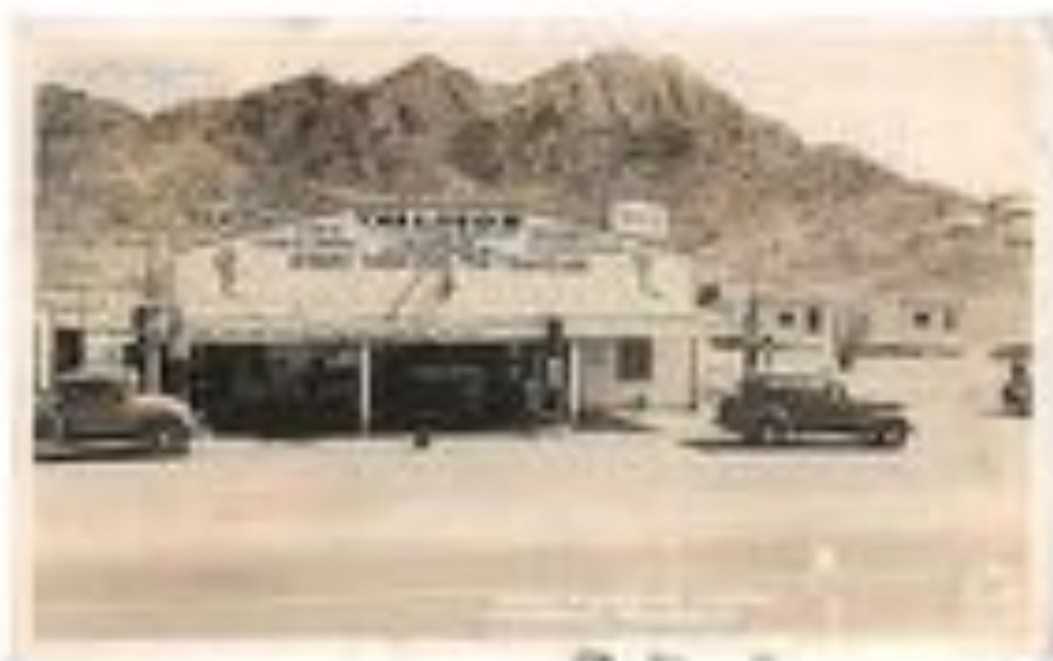
Gas Station, 1930s
